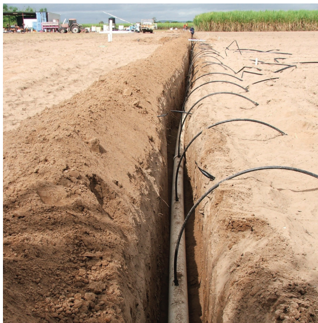
Above: Drip tape being installed. Photo courtesy of Steve Attard.
